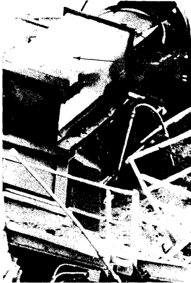
Closer view of the explosion damage and distortion of the belt conveyor section on the coal bin.
